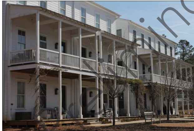
The Docks envisions diverse residential opportunities, including townhouses with a complimentary character.
