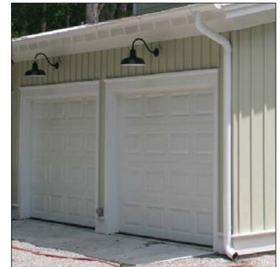
Wall-mounted lights at garage doors
