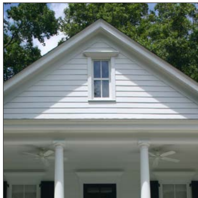
Frieze board at rakes and eaves
