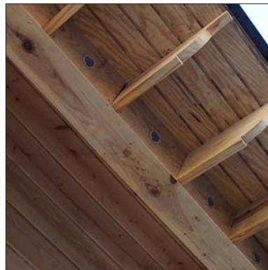
Discreet vents in open eave
