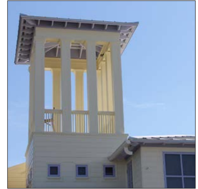
View tower above top story
