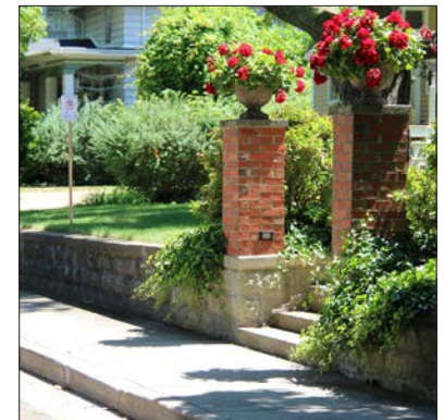
Retaining wall with entry piers
