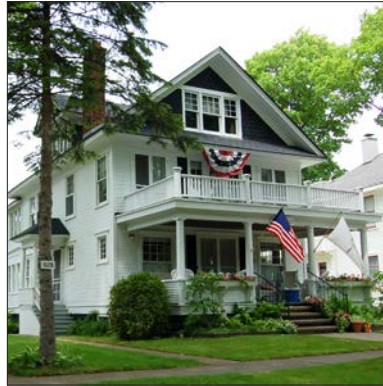
Third floor within gable roof front
