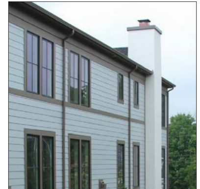
Stucco chimney with projecting cap
