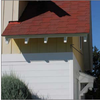
Open eave with rafter tails
