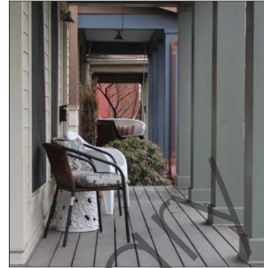
Low porches with no railing
