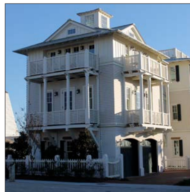
Balconies at second & third floors
