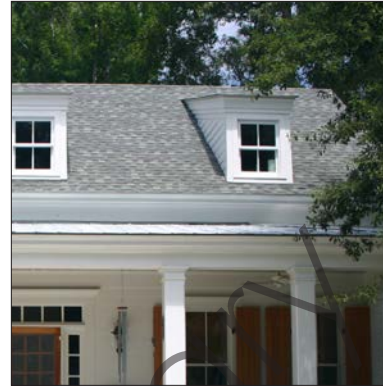
Shingles on main roof, metal on porch
