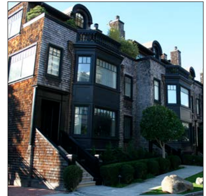
Stepped roof terraces
