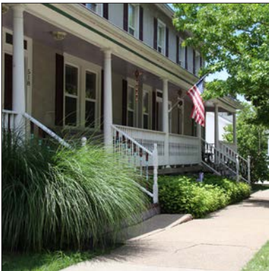
Close porch softened by plants
