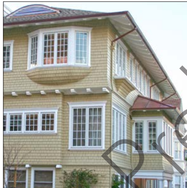
Distinct bay roof under deep eave.
