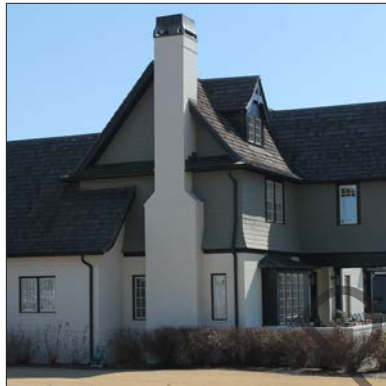
Masonry first floor & chimney
