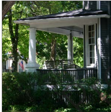
Ogee gutters must return into wall
