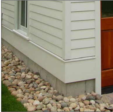
Concrete base & water table
