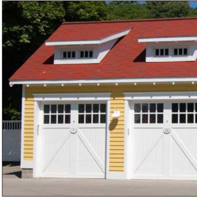
Carriage doors where required
