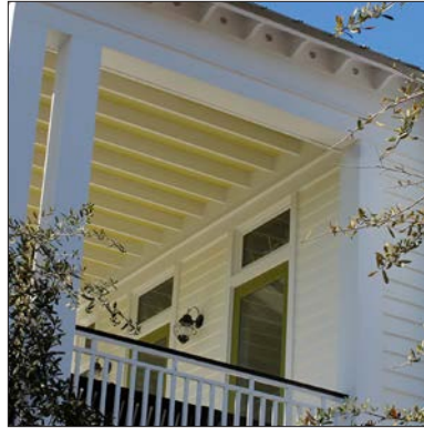
Lap siding finished with wide casing
