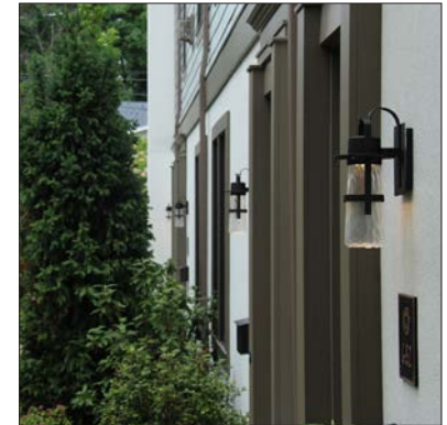
Wall-mounted lights at entrances
