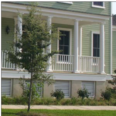
Stucco porch piers
