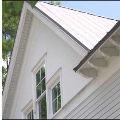
Soffit material appears as wood
