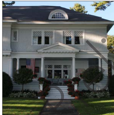
In-board porch within main massing
