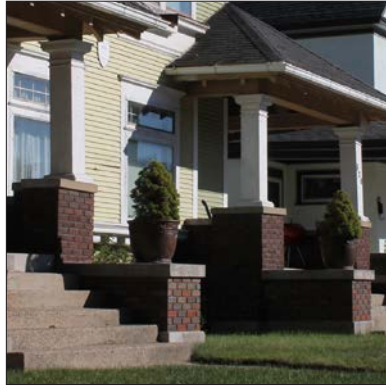
Brick base with siding above
