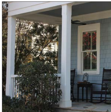
Porch ceiling above beam
