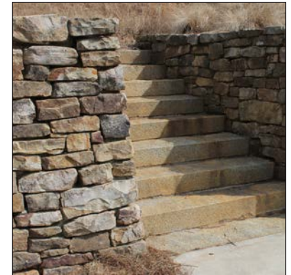
Tall retaining wall
